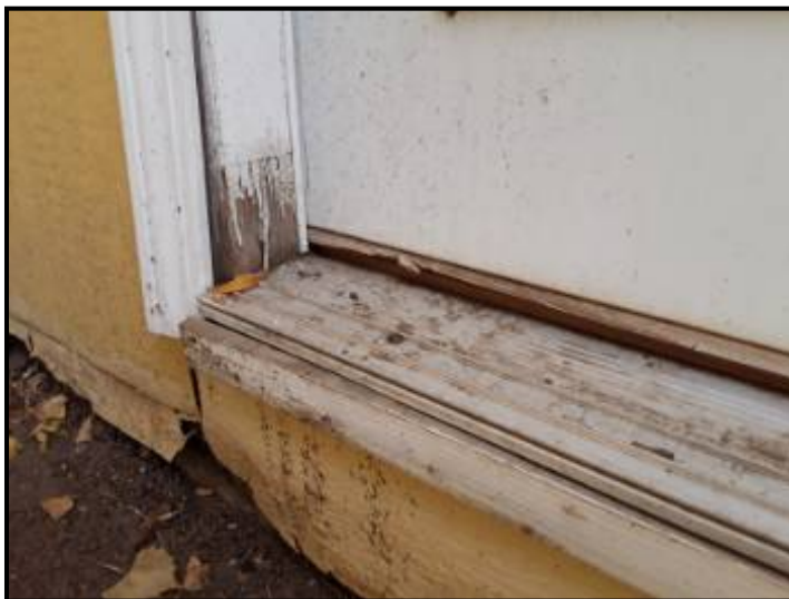
Peeling paint observed, suggest scraping and painting as necessary.
