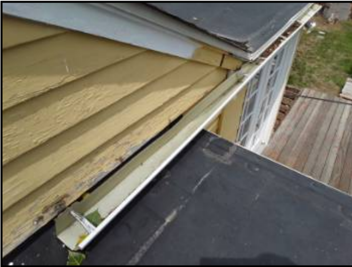
Sagging gutter, detached from building.
