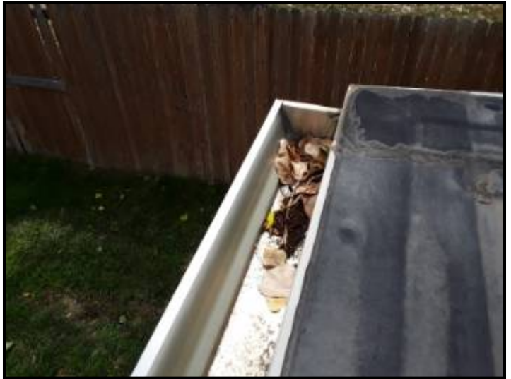
Debris in gutters.
