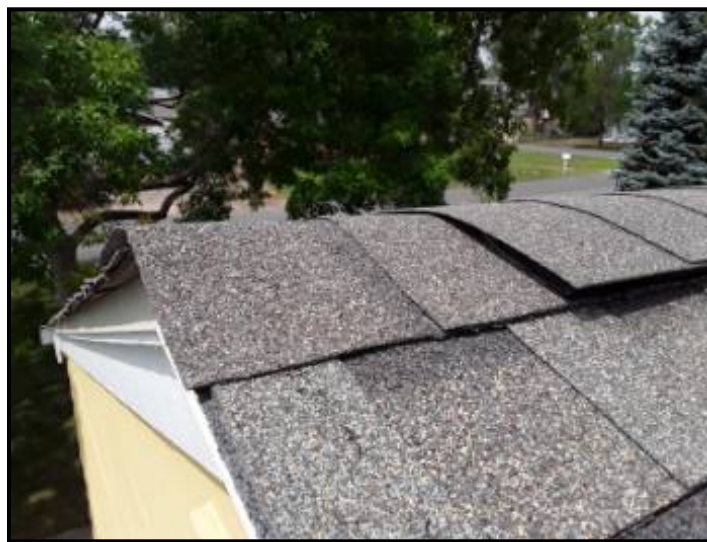
Improper ridge vent installation.
