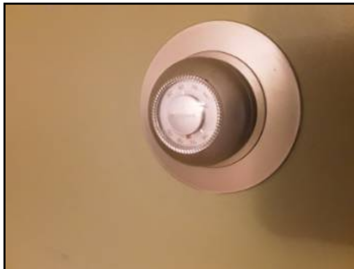
Analog, non-programmable type.
