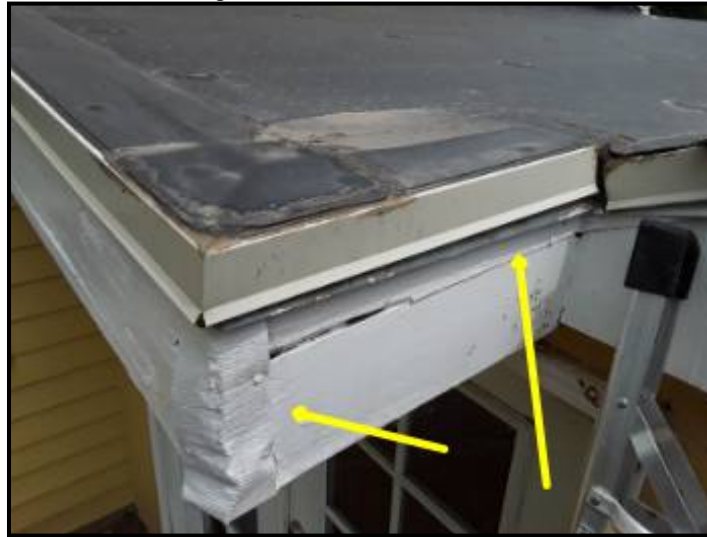
Missing gutter causing rotting fascia.
