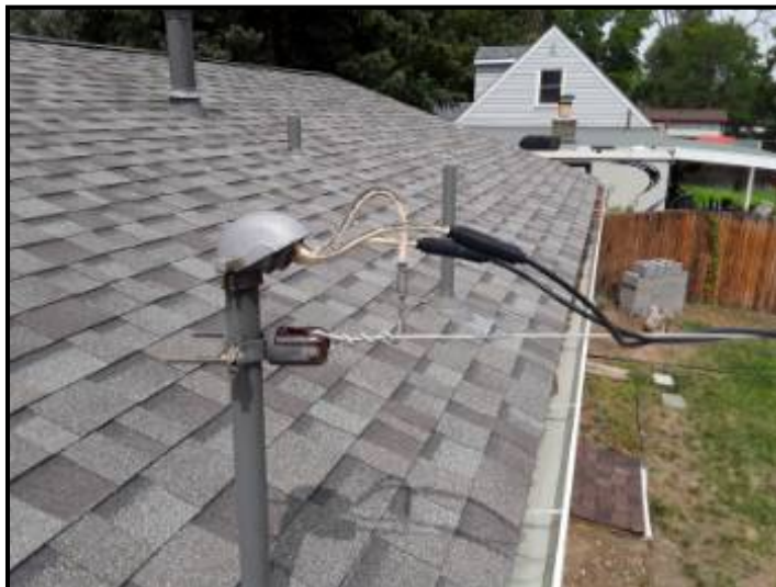
Missing drip loop.
