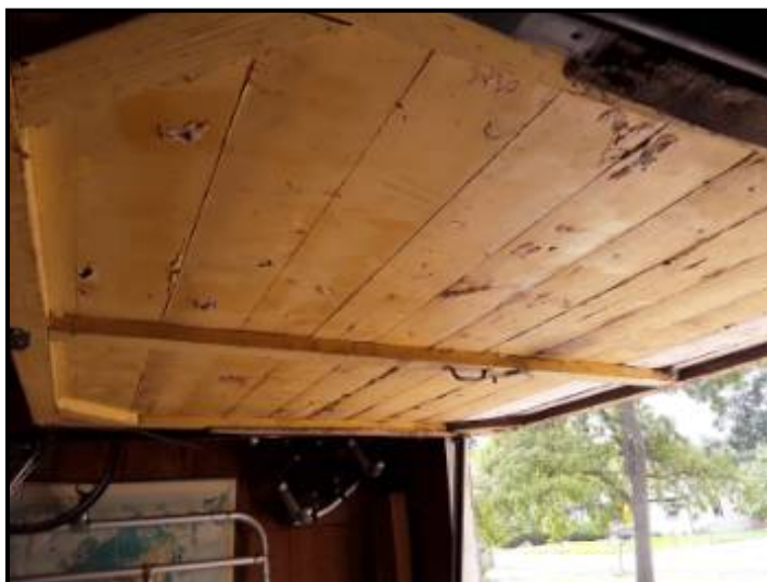
Rotted wood at overhead door. Recommend repairing damaged areas.
